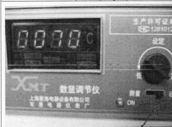
Photo 15. Safety oil temperature preset
